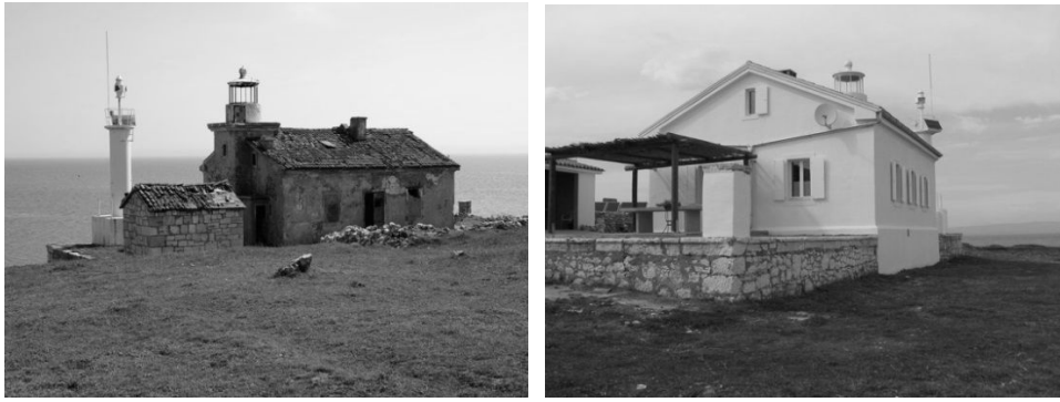
Picture 6: Marler Lighthouse, Republic of Croatia - before and after renovation
